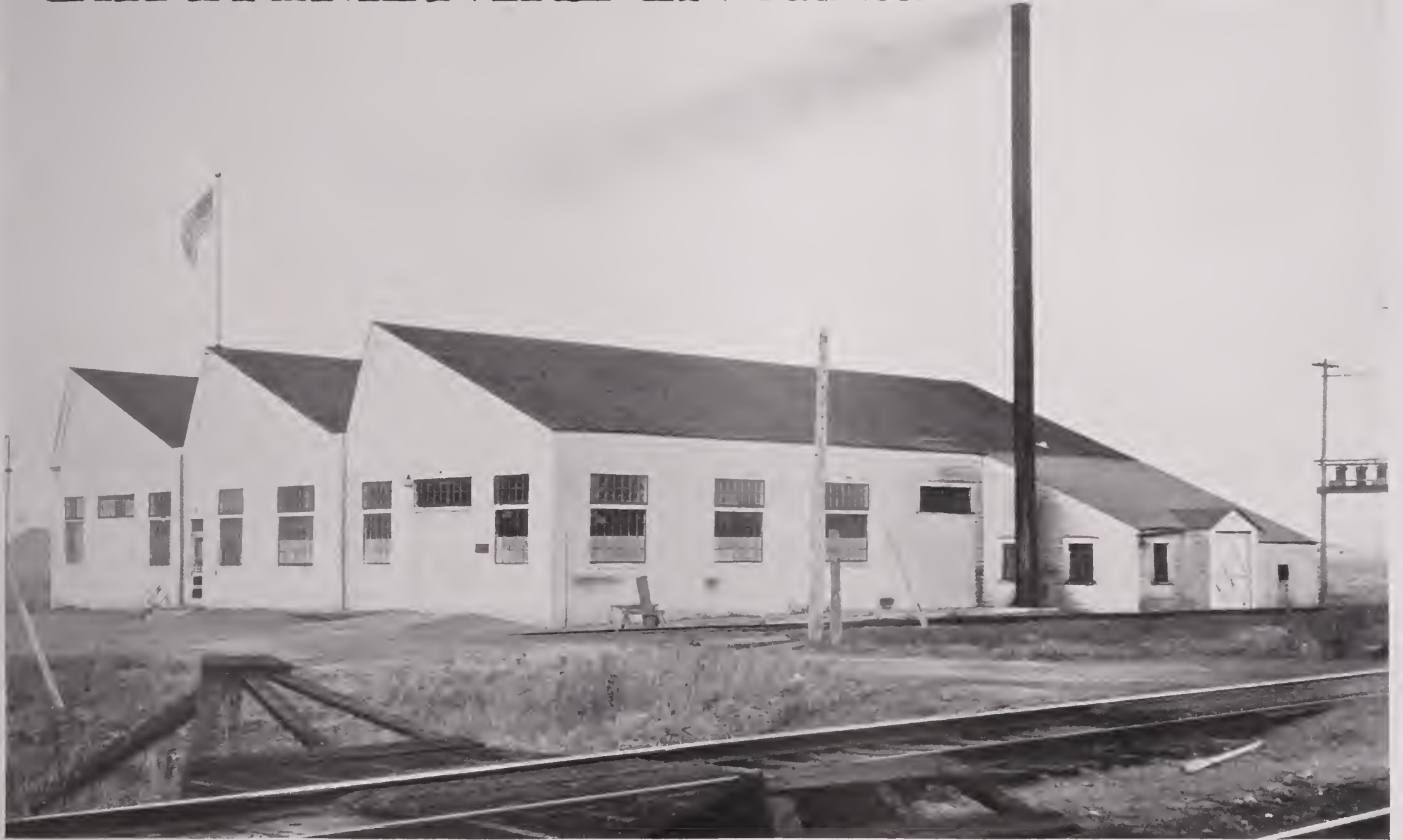
FIRST UNIT OF PAN PLANT
